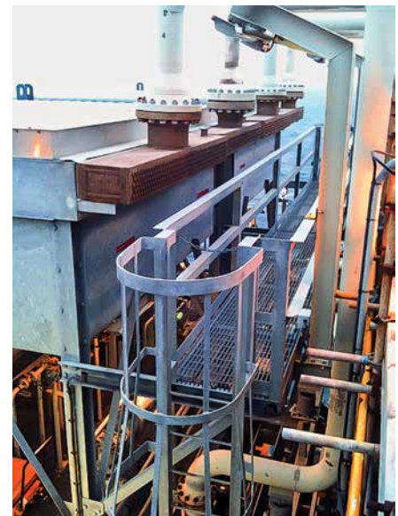
Fig. 2. One of the likely leak areas is a fin fan cooler.
